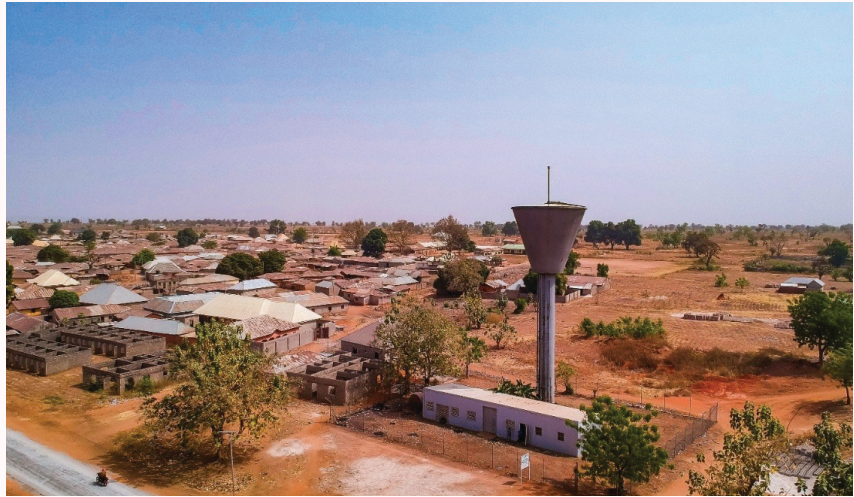
^ Kataeregi Water Scheme – One of the water infrastructures rehabilitated with the support of UN-Habitat in Niger State. © UN-Habitat/Emmanuel Adeleke
